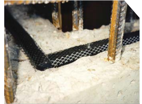
Waterstop RX101® is a sodium bentonite based waterstop designed to stop water infiltration through cast-in-place concrete construction joints.
