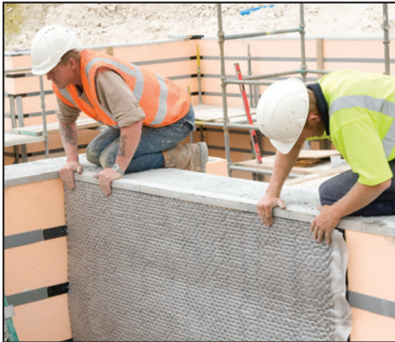
Fig 1: Position Membrane
