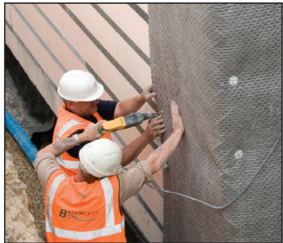
Fig 4: Fixing Membrane around corner
