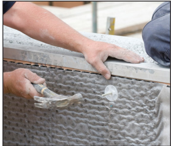
Fig 2: Fix Membrane
