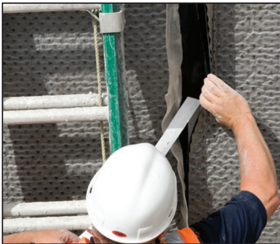
Fig 3: Tape Joints
